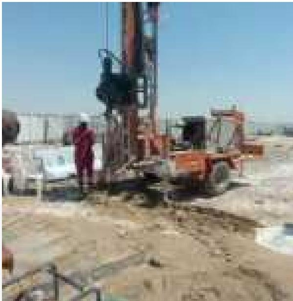
The Al Shamkha Future School project involved a comprehensive geotechnical and hydrological study to evaluate subsurface conditions and decrease the ground water level at the project site, groundwater behavior, and associated challenges for the development. The investigation included drilling boreholes, conducting permeability tests, pumping test, geophysical surveys, and monitoring groundwater levels.
