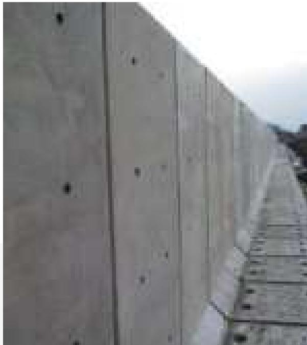
SAC successfully completed the "Road Safety Enhancement" project in Abu Dhabi City. The project aimed to design and implement a retaining system to protect the road infrastructure from potential hazards posed by adjacent embankments and future developments. The focus was on ensuring road stability, enhancing safety, and mitigating risks of embankment instability.
