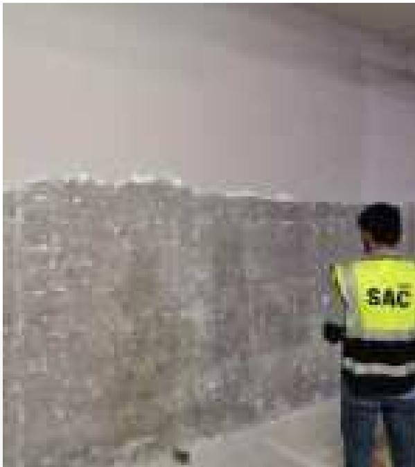
SAC was engaged by The First Group to investigate significant water leakage in the basements of the Diamond Tower. The basements showed concrete deficiencies, including peeling paint, corroded steel, and spalling surfaces due to water seepage. The investigation aimed to assess the condition of the concrete and determine the root causes of these defects to propose effective repair methodologies.
