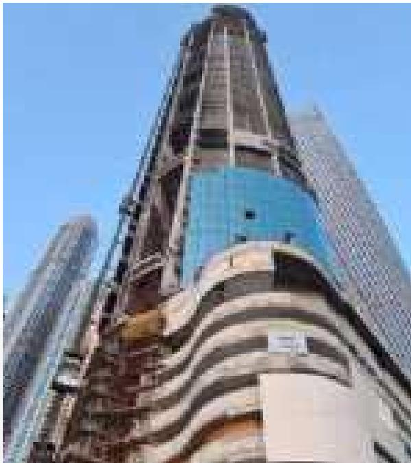
SAC was appointed to analyze the structural impact of the Ciel Tower's deep foundation and shoring systems on the surrounding infrastructure, including the MARINA Bridge, the adjacent RAMP retaining wall, and the Canal Quay Wall. Continuous settlement, movement, and active cracking were observed in the surrounding area during construction, affecting the MARINA Bridge and nearby utilities.
